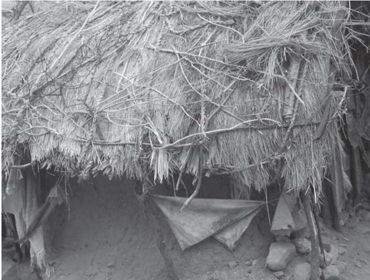
The dilapidated house of a fluorosis affected family in Tutu Sahi of Boudh district
